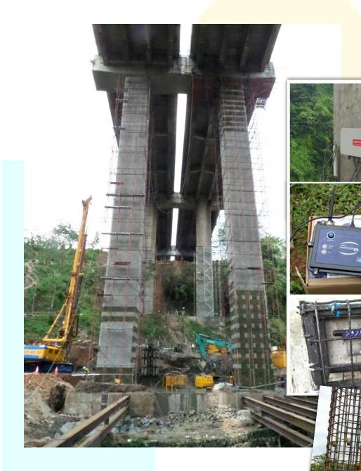
TiltMeter, Inclinometer, Piezometer, Vibrating Wire Strain Gage
